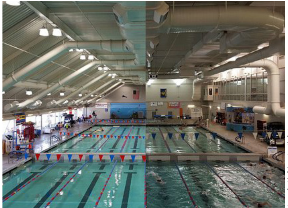
Before (right) and after (left) photograph of pool with LED lighting.
